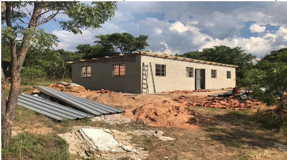
Molokomme new house under construction.
